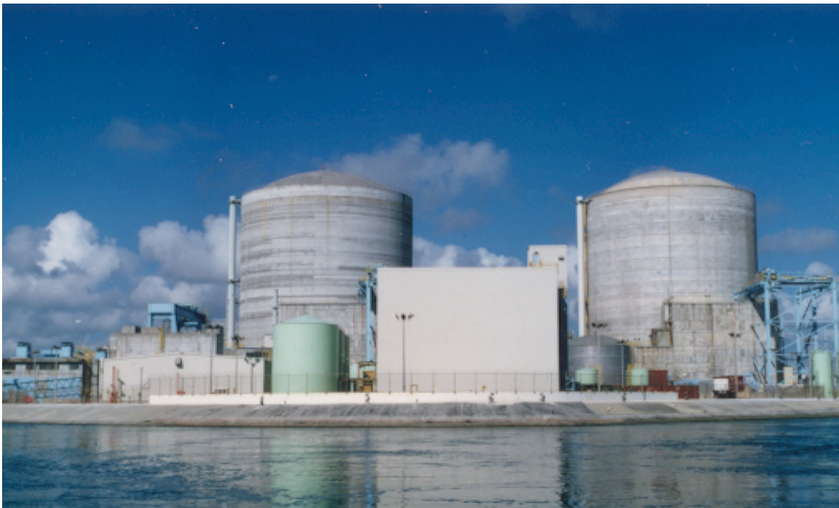
St. Lucie nuclear units 1 and 2 (Florida, USA) are cooled using large water intake canals; most thermoelectric plants rely on massive canals or pipes to supply their below-market cooling water.
